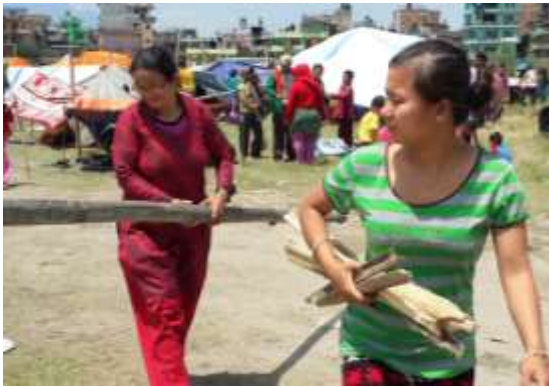
Fig 9 Salvaging materials from destroyed buildings
