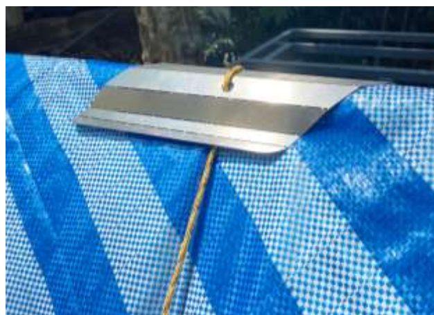
Fig 21 Clamp over shelter frames
