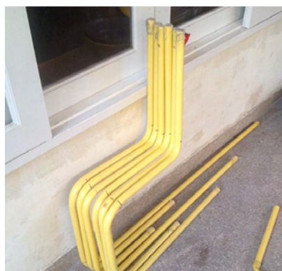
Pic 2. Using heat to bend the pipes.
